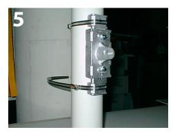
Install second banding strap on bottom of back plate and tighten down.
