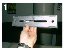
Insert stove bolt from behind through elongated slot and hold in place.
